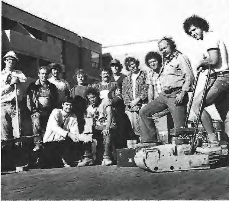
The Paving Stone Installers
